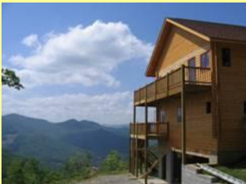
NEW HOME UNDER CONSTRUCTION IN THE SANCTUARY MTN GROVE
